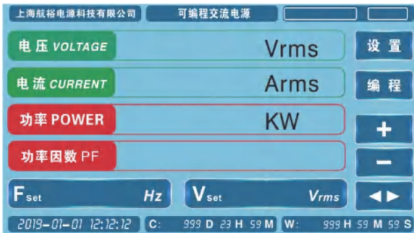
Single phase power supply main interface
